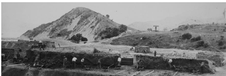
Tokomaru Bay freezing works under construction.
